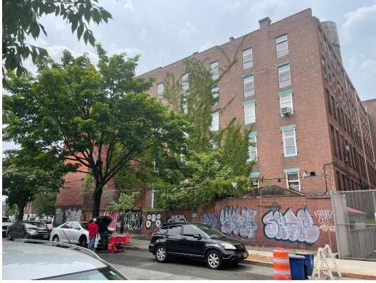
Figure 2. View of the abandoned building and lot from 440 Canal Pl
